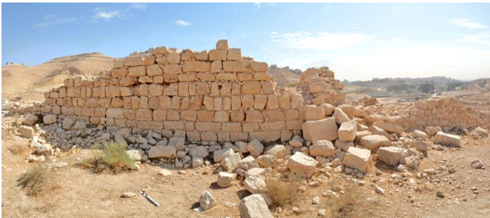
Fig. 3 - The collapsed south-eastern corner and the eastern wall of the khan.
