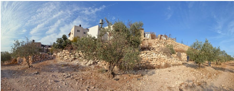
Fig. 47 - Modern terrace wall overlapping the Iron Age fortifications at Khirbet el-Kôm.
