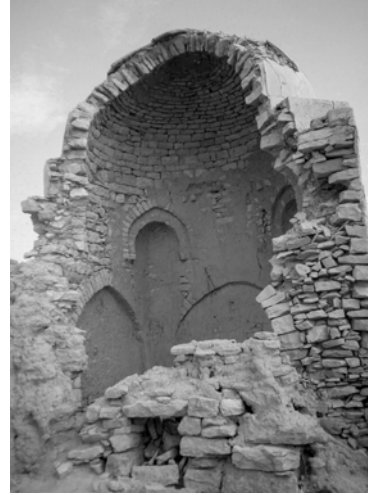
Fig. 5 - Barāqish. The chahār ṭāq mausoleum, west half: the interior, showing walled-up doorways, squinches and the dome (© M.V. Fontana 1992).
