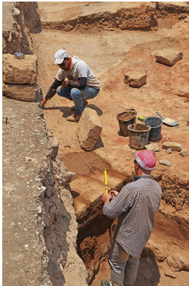
Fig. 16 - Restorers preparing the mortar bed for the sacrifice layer of new bricks.
