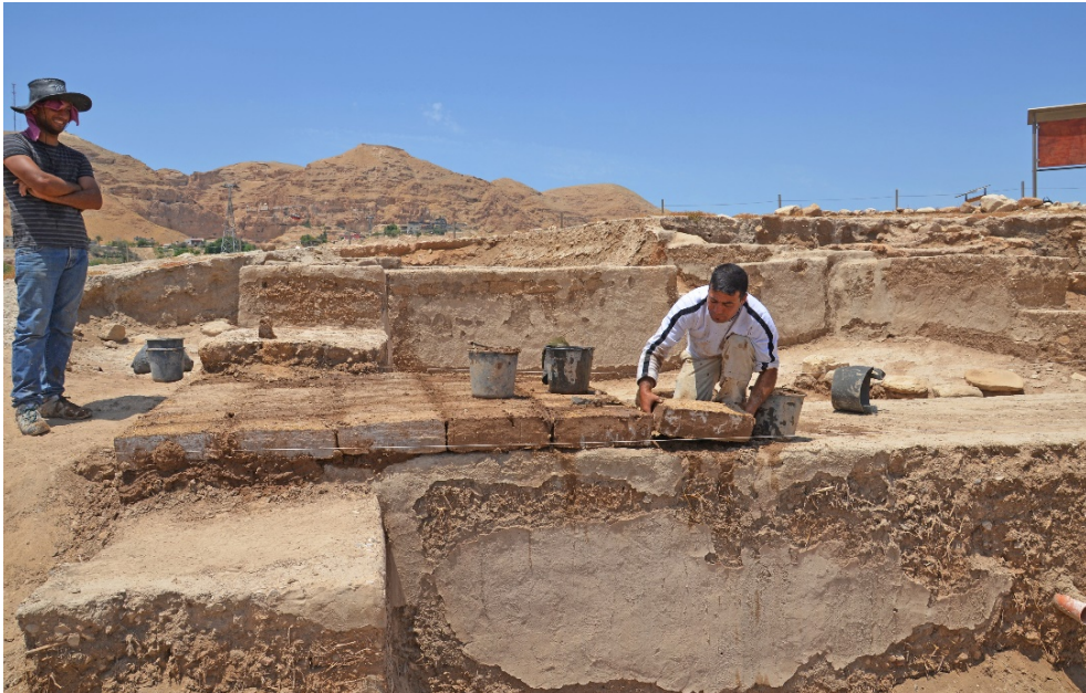
Fig. 21 - Training of a restorer laying bricks on the main wall of Palace G.
