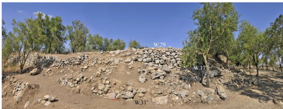
Fig. 29 - Walls W.29+W.39 and W.31+W.17, at the western edge of Acropolis in Area C, seen from west.
