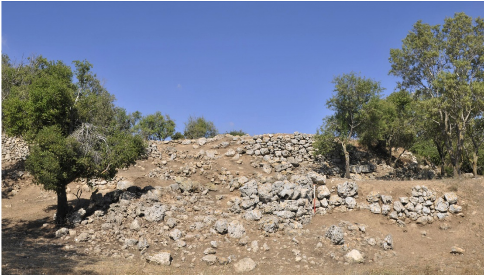
Fig. 30 - Tower T.25 in Sector XIII seen from the west.
