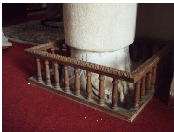
Fig. 2 - A 6 th century capital re-used as column basis in Deir el-Hammām (photo P. Buzi).
